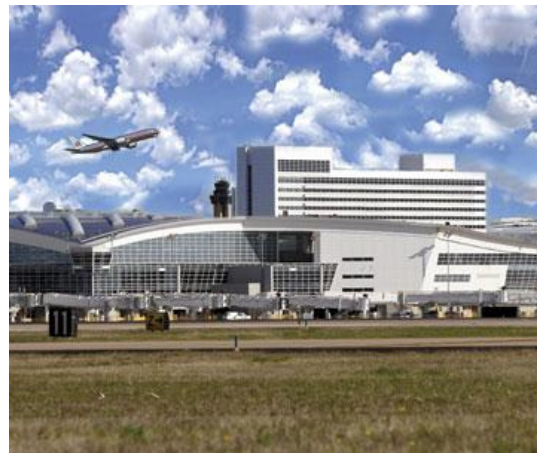
Airside with plane on Terminal D at DFW.
